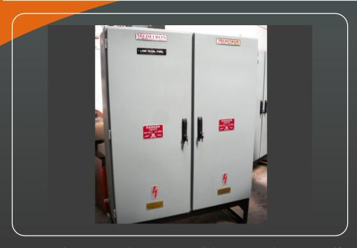
The MEDITRON make Crane Control Panel comprise all the power switch gear required for crane control except power resistors which are separately fitted. The operator's control & Arm chair unit is also separately supplied.
