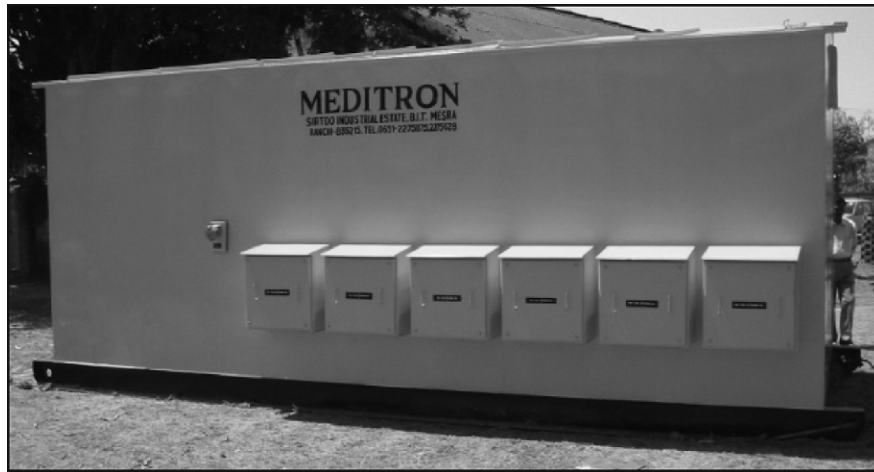
Hut Type 20 MVA Substation
